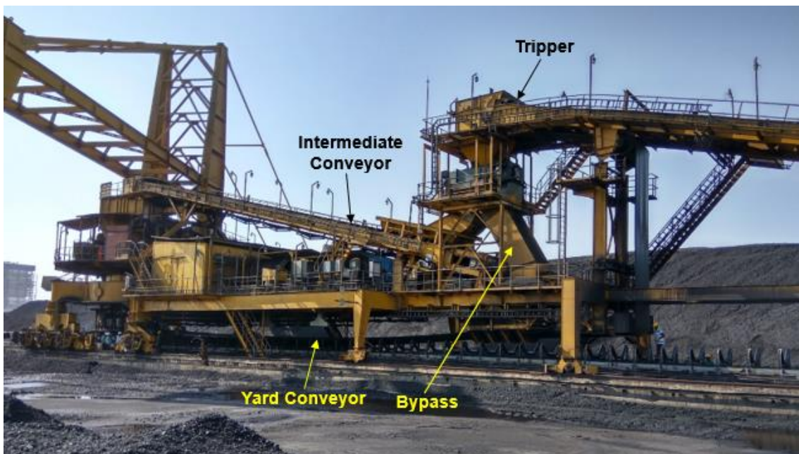
Stacker cum Reclaimer with Intermediate Conveyor for Bypass - Close Up View
