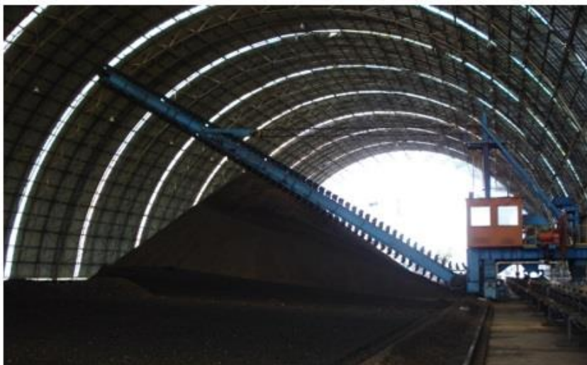
Photograph of Side Scraper Reclaimer
