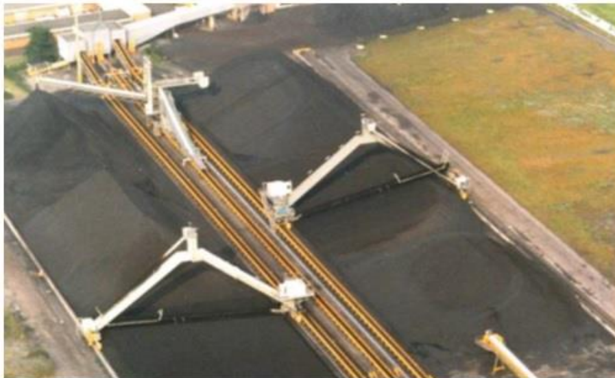
Stockpiles on Both Sides of Luffing and Slewing Stacker
