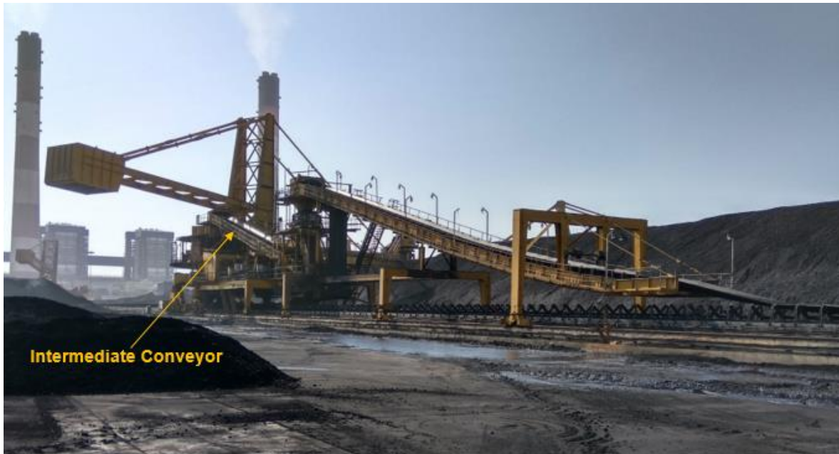
Stacker cum Reclaimer with Intermediate Conveyor for Bypass
