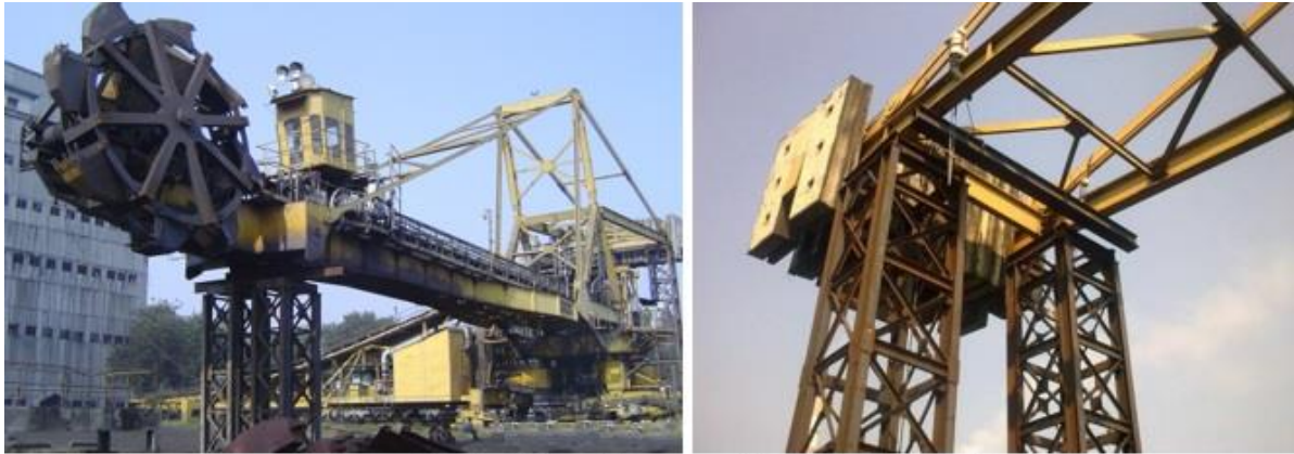
Supporting of Bucket Wheel Boom and Counter Weight Boom
