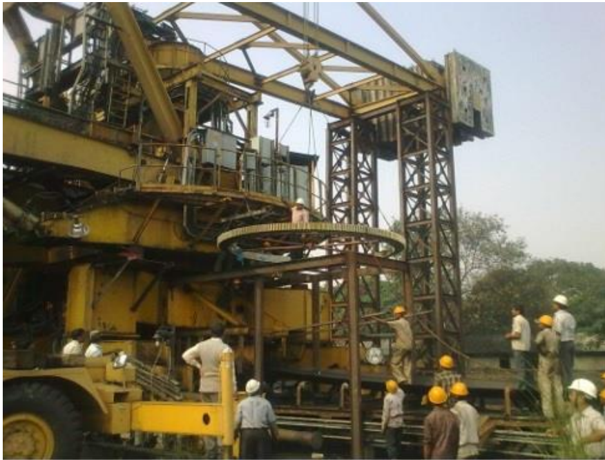
Replacement of Slew Bearing
