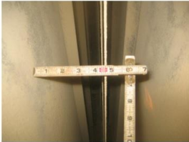
Misalignment Between Discharge and Collection Electrodes
