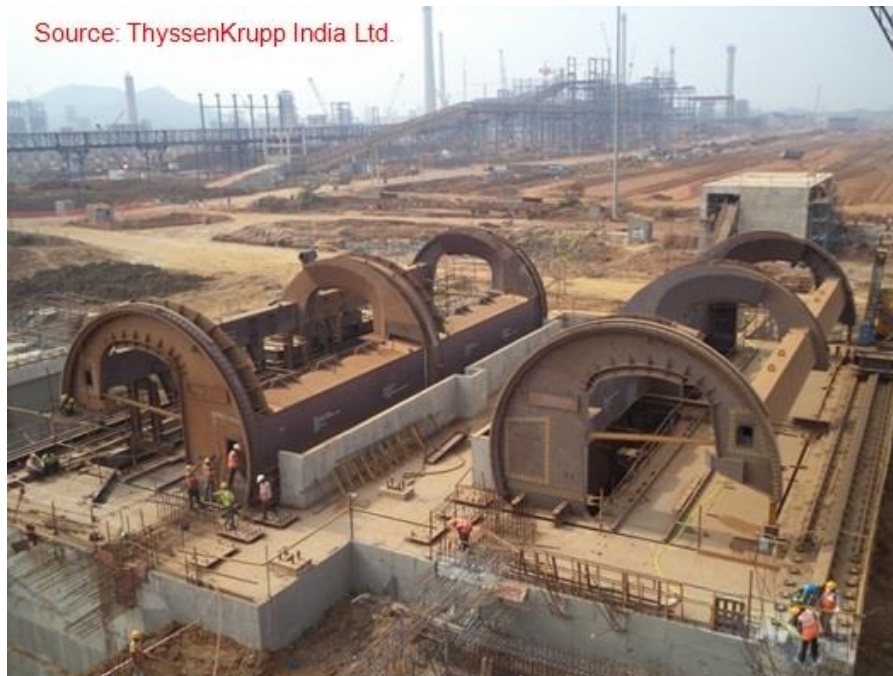
C-type Rotary Tandem Wagon Tippler
