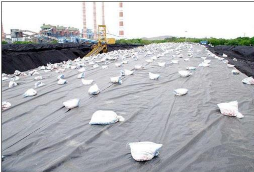
Covering of a Pile by LDPE Sheets
