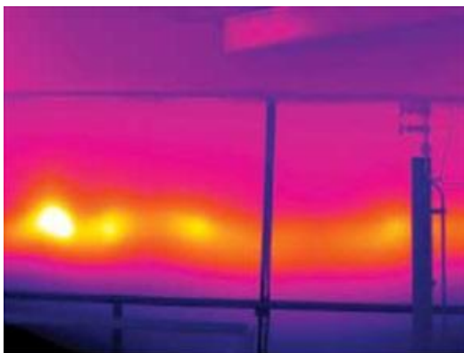
Infra-Red Image of PRB Coal Silo Fire
