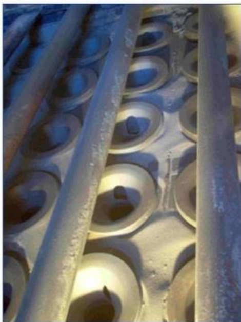
Misaligned Blow Pipe and Filter Bags
